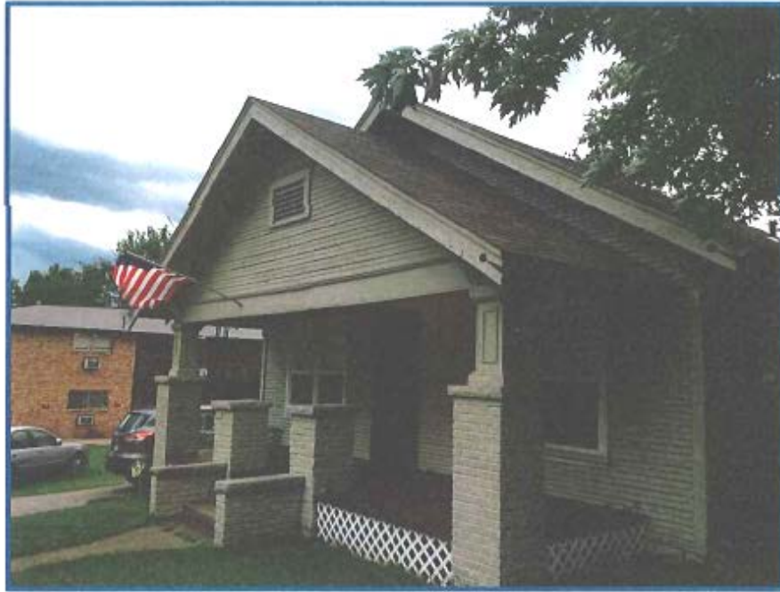
West Elevation of Residence/Office
