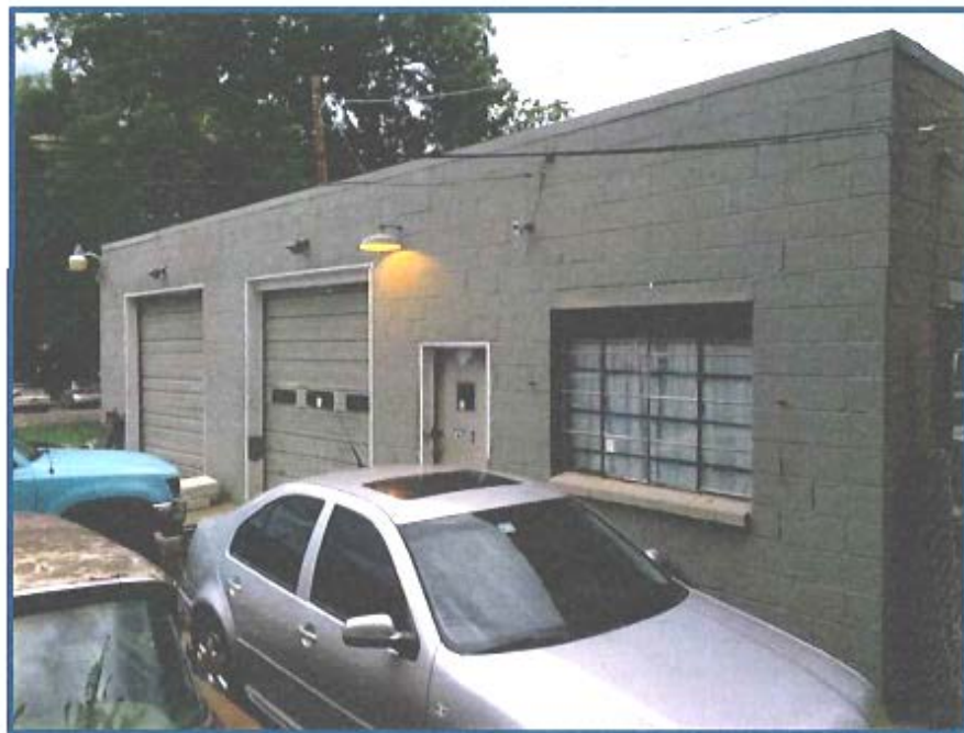
West Elevation of Shop/Warehouse
